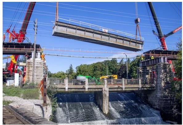
Crews from Mammoet carefully swing the largest span of Allan's Bridge into position over the Speed River. September 26, 2021. Jacob Patterson Photo.
